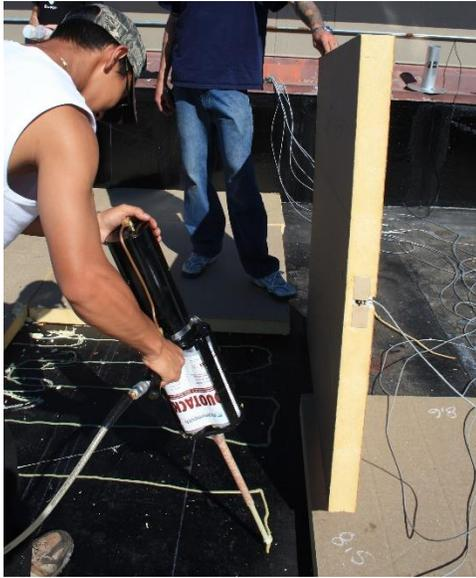
*Figure 3.10 Study insulation board immediately prior to being adhered to air and vapour barrier on top of roof deck.*
