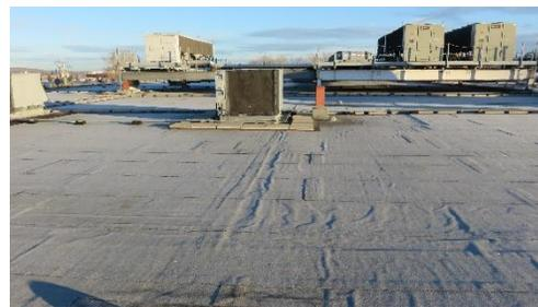
*Figure 2.2 Distortion of 2-ply SBS roofing membrane in a conventional roof assembly with polyiso insulation.*
