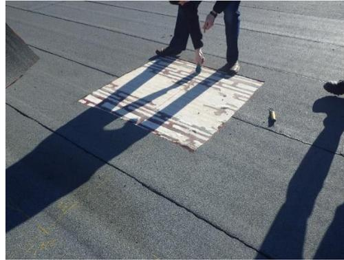
*SBS membrane removed in order to observe dimensional change in polyiso as well as its overall condition.*
