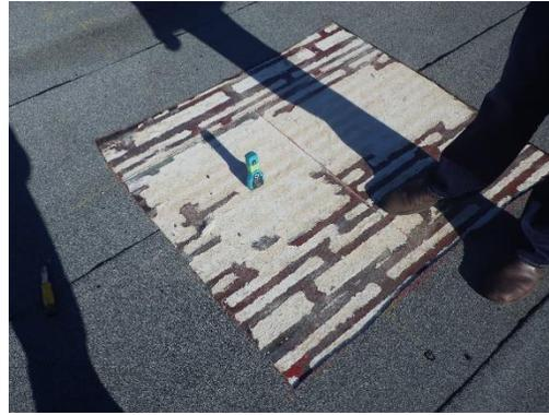
*Figure 3.22 Overall shot of 4'x4' exploratory roof opening.*
