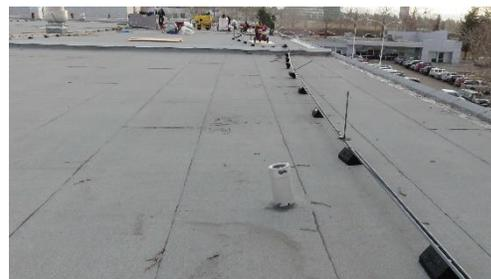
*Figure 2.4 Damage to roof stack vent likely due to movement of underlying polyiso insulation.*
