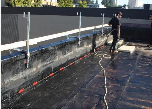
*Roof assembly constructed up to vapour barrier. Wiring for sensors during installation.*
