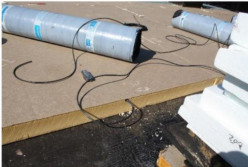
*Figure 3.8 RH and temperature sensor during installation, installed into top surface of polyiso insulation. Typical of all RH/Temp sensors.*
