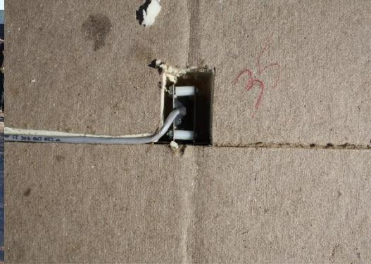
*Displacement sensor installed with metal contact plate in polyiso roof insulation. This is typical of how all displacement sensors were installed.*
