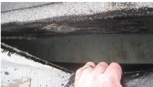
*Figure 2.3 Observed 3"+ Gap between parapet and insulation likely due to dimensional movement and shrinkage of polyiso insulation.*
