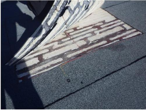
*Figure 3.21 SBS roofing membrane being removed in order to visually inspect polyiso insulation*
