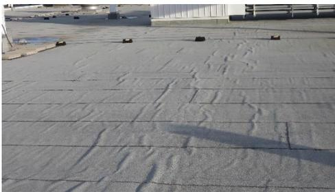
*Figure 2.1 Wrinkling and distortion of 2-ply SBS roofing membrane in a conventional roof assembly with polyiso insulation.*
