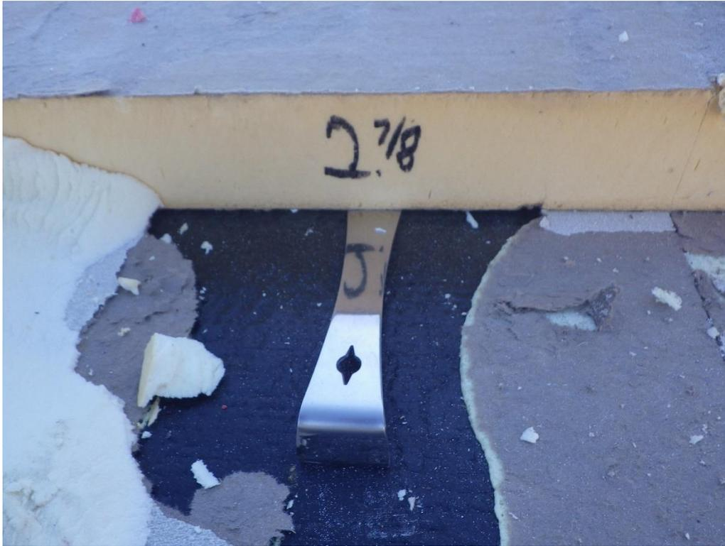
*Figure 3.25 Polyiso insulation board thickness, measured at factory edge. Several of the exposed insulation boards appear to have shrunk in thickness during the course of the monitoring study, from 3" initial as purchased to 2 7/8" in-service.*
