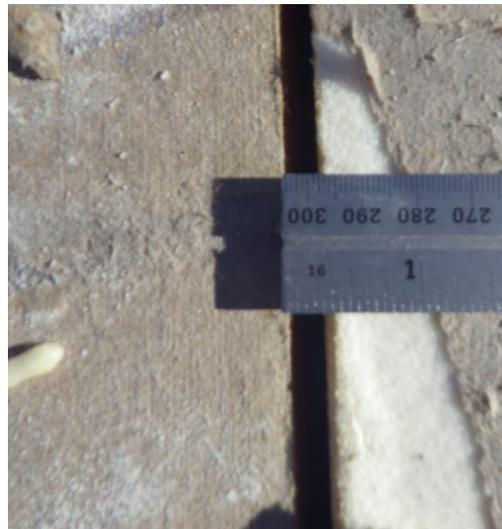
*Figure 3.24 ~5mm gap observed between edges of polyiso insulation boards.*
