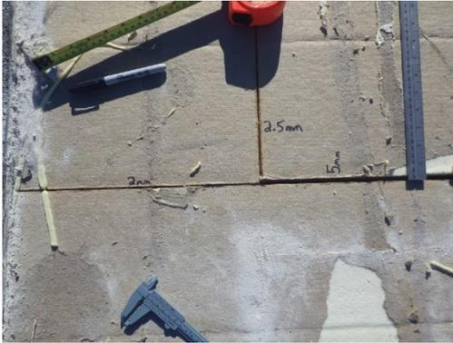
*Gaps between polyiso insulation boards, ranging from 2mm - 5mm. These measurements generally confirmed the accuracy of displacement sensor readings.*
