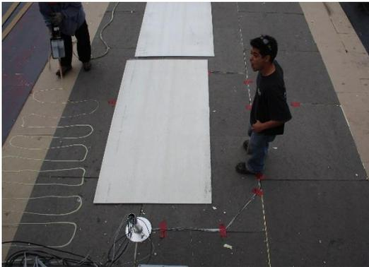
*Protection board immediately prior to installation onto exterior surface of polyiso. Note the adhesive being applied.*
