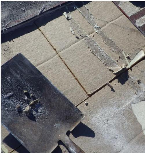
*Figure 3.23 Polyiso insulation board exposed during exploratory roof openings.*
