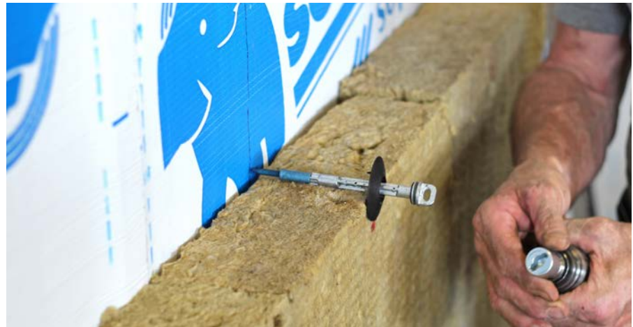
Masonry ties installed through exterior insulation
