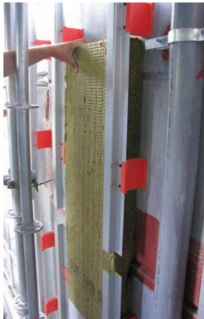
Insulation upgrade to the Belmont Building in Vancouver.
