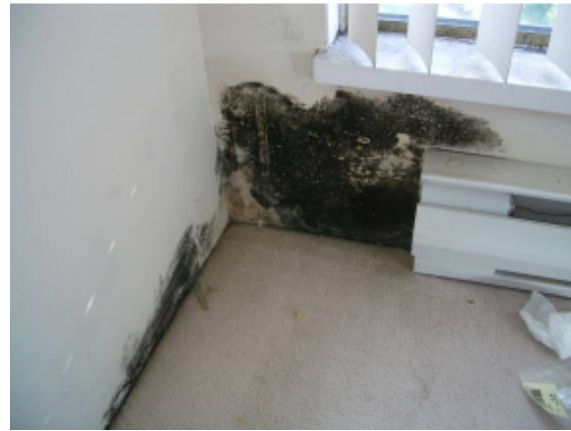
Figure 6: Fungal growth on the interior finishes below a window at an exterior wall.
