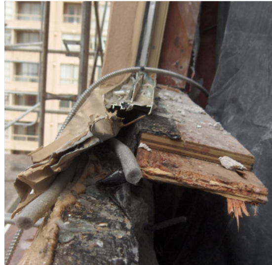
Figure 4: Cut section of a window sill at impact location
