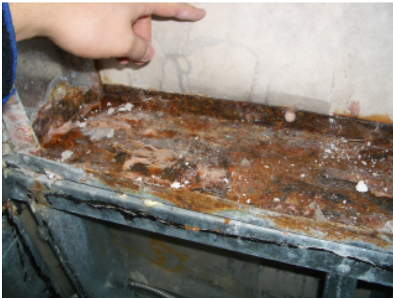
Figure 5: Corrosion of the exterior wall steel studs and deterioration of the exterior gypsum sheathing
