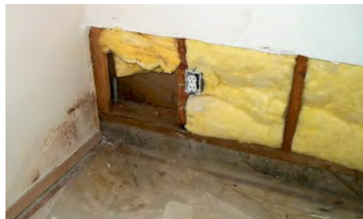
Figure 9 Insulation and Studs in Good Condition on Exterior of Vapour Barrier
