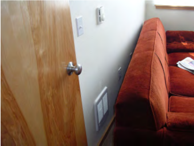
Figure 3 Undercut door intentionally blocked to resist drafts and control odors from hallway into suite.
