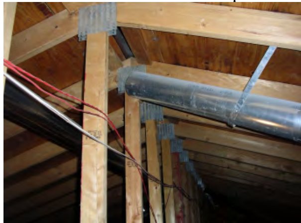
Figure 6 Exhaust duct terminated in attic space.
