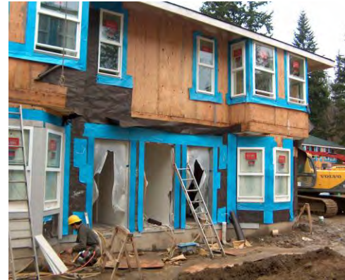
Excessive and improper use of vapour-impermeable, self-adhered membrane (blue) around windows and other penetrations of a wood-frame building in Climate Zone 5.
