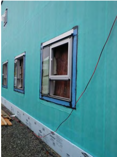
At this 3-storey wood-frame recreational building, self-adhered vapour-permeable membrane is applied directly over plywood to form the air-barrier system. Self-adhered membranes may improve detailing and provide a more rigid and durable air-barrier system than sheet applied and taped membranes.
