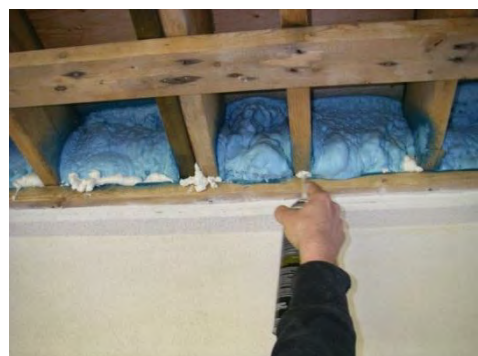
Polyurethane spray foam is used as a transition air-barrier material to seal and insulate the space between roof and floor framing. The use of spray foam to fill small to large gaps in conjunction with other air-barrier strategies is common.
