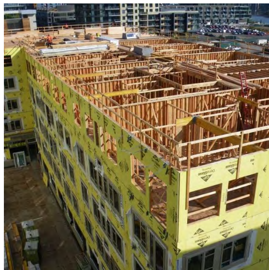
Construction of a 6-storey MURB with non-combustible gypsum sheathing. Framing factors at lower floors are higher than at upper floors in order to accommodate structural loads. The effective R-value of these walls will be affected by this wood-framing factor and the chosen insulation strategy.
