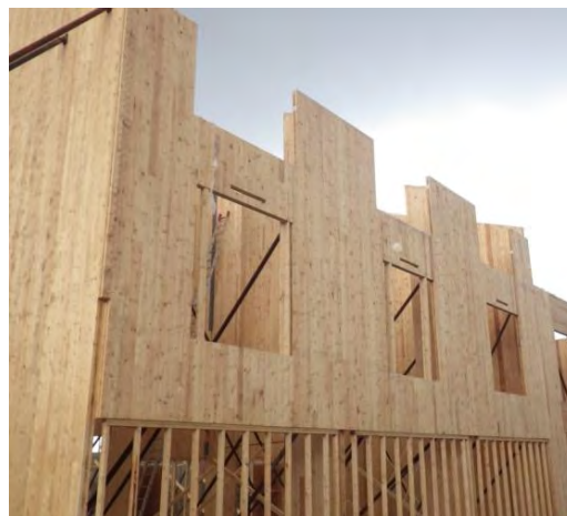
Large CLT wall panels make up most of the structure of the building and provide a substrate for the water resistive barrier and exterior insulation.
