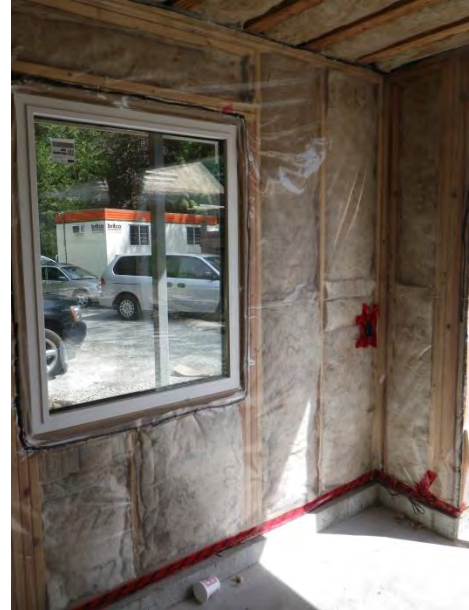
The sealed polyethylene approach uses acoustic sealant and red tape for details and transitions, such as in this wall around the window and light switch. Because the industry is familiar with this approach and the combined vapour barrier function, many designers will elect to use this approach in designs.
