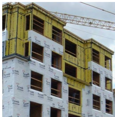
An exterior air-barrier approach can be utilized to either seal the joints in the exterior sheathing (gypsum in this MURB) or seal the exterior sheathing membrane (SBPO in this MURB). Selection of which component to seal will depend on cladding type, MURB height, and the contractor's familiarity with the approach.
