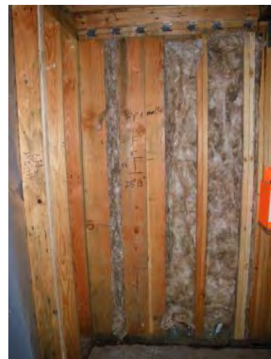
Fibreglass insulation placed between wood framing in a 5-storey MURB under construction. The effective R-value of the wall assembly is much less than the R-20 nominal batt insulation due to thermal bridging of framing, particularly when heavy timber elements are used at lower floors.
