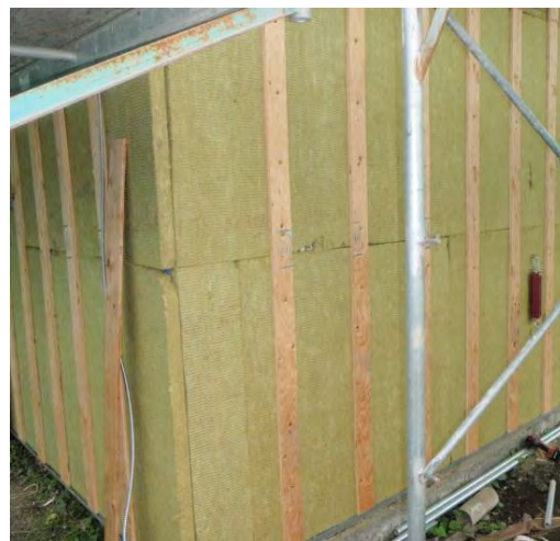
Split-insulation wall assembly consisting of rigid mineral fibre on the exterior of the wood sheathing and sheathing membrane. Cladding will be attached to the vertical strapping on the exterior of the insulation, which has been fastened back into the structure using longer screws.
