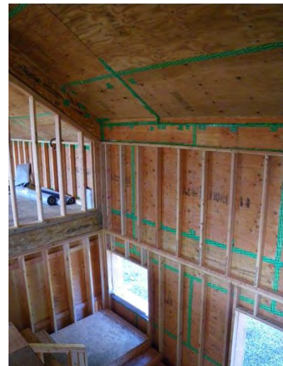
A rigid, interior, air-barrier approach using taped plywood sheathing at the inside of the wall assembly is common in Europe and many Passivhaus designs with highly insulated wood-frame walls (pre-fabricated and site built).
