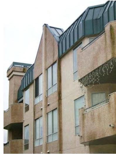
The lack of appropriate protection of the face seal stucco walls and poor interface detailing have resulted in the deterioration of many wood-frame building enclosures in wet climate zones.
