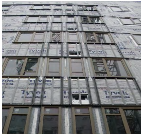
There is very little test data available to allow for a more analytical or even empirical approach to determining the structural adequacy of sheet-membrane barrier systems. Precautionary measures could include tightly spaced strapping to secure the membrane, and selection of more robust membranes (i.e., in terms of strength and tear resistance). The use of self-adhered and liquid-applied membranes basically makes the sheathing and membrane an integral, rigid, air-barrier material.
