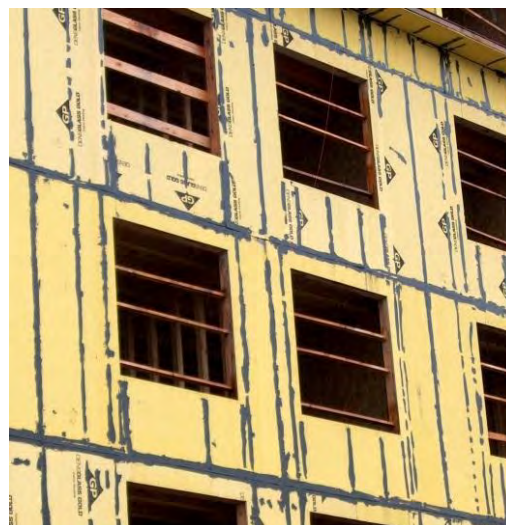
The exterior, sealed-sheathing, air-barrier approach is a rigid and durable strategy for a wood-frame MURB that meets the five requirements for an air-barrier system.
