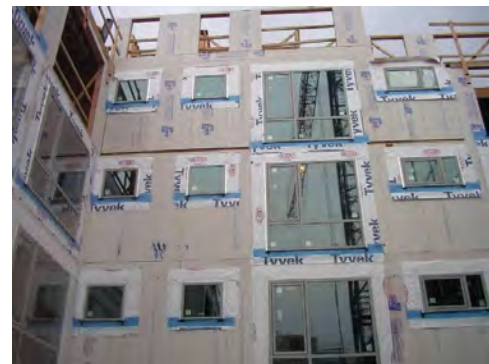
Minimal and proper use of impermeable, self-adhered membrane (blue) at window sills, with vapour-permeable membrane used at the jambs and head of the windows of a wood-frame MURB in Climate Zone 4. Window detailing is covered in further detail in Chapter 6, complete with build-slides that show sequencing of this detail.
