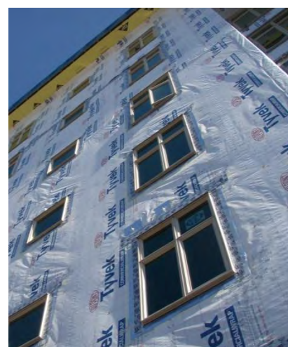
When properly detailed and supported during construction and in-services, the exterior, sealed sheathing membrane, air-barrier approach can be a successful strategy for air-flow control in a MURB.
