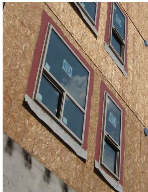
Liquid membrane used in the window rough opening to simplify sequencing and detailing.
