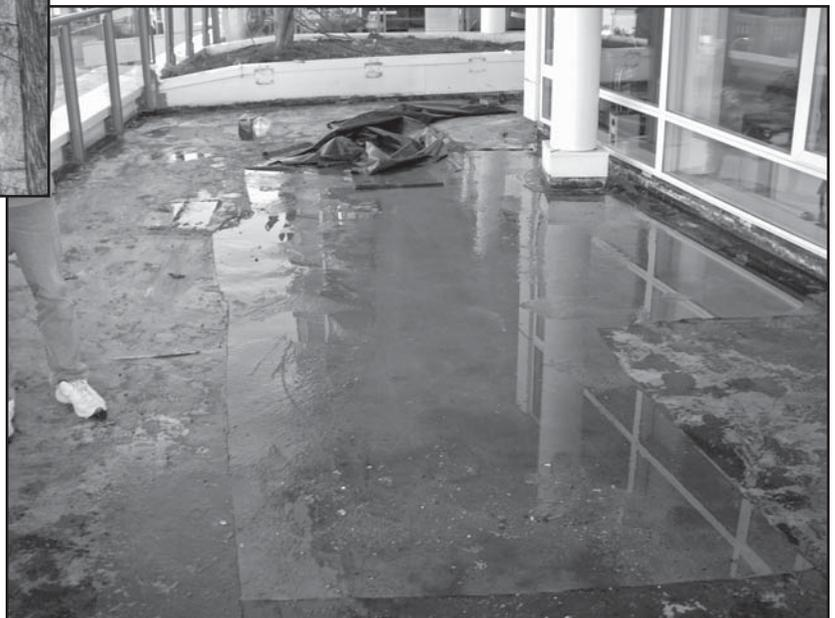
**Figure 4 – Water beneath blistered membrane over entire deck.**
