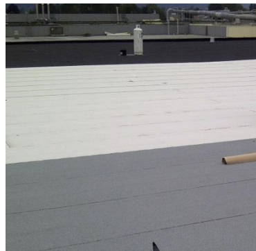
Figure 5 Membrane Cap Sheet Colors (Reflective White, Grey and Black) Shown on Left in Lab (Un-soiled and New) and Right in Field Shortly After Installation.
