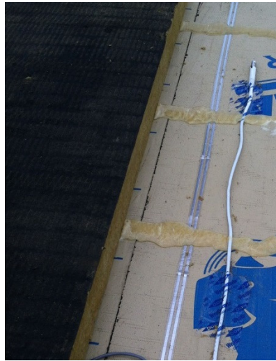
Figure 7 Moisture detection tape (left) and RH sensor (right) above air/vapour barrier below insulation. Note also the ribbons of adhesive.
