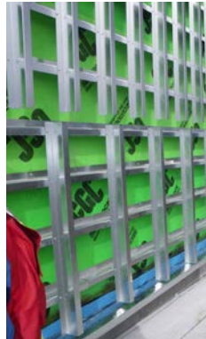
Figure 6: Crossing Z-girt assembly consisting of horizontal and vertical Z-girts attached at crossing points.
