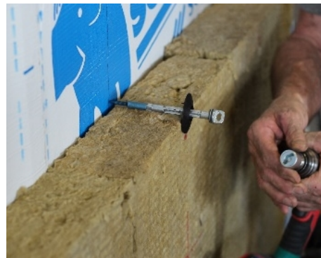
Figure 16: Examples of some different masonry ties installed through exterior insulation.
