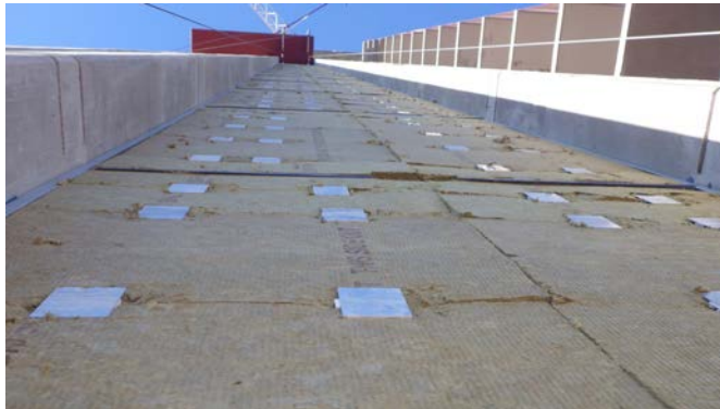
Figure 22: Example of insulation retained by intermittent cladding support clips behind metal panels. The metal panel support structure overtop will further retain the insulation in the assembly here.
