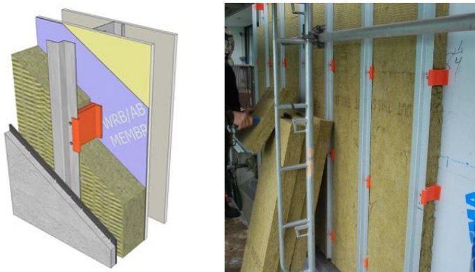
Figure 13: Fiberglass clips with vertical Z-girt attached with screw fasteners through the fiberglass clip into the back-up wall
