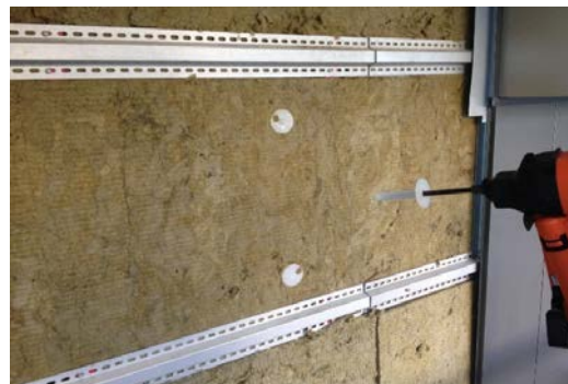
Figure 24: Example of plastic fuel-cell actuated insulation fasteners installed after insulation and girt system is installed to retain the insulation.
