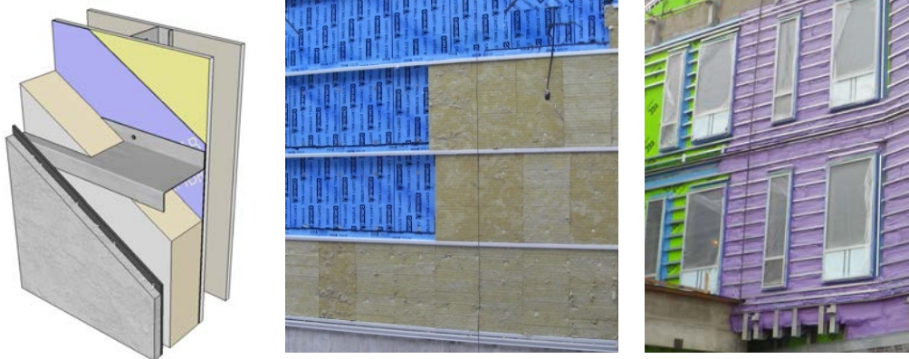
Figure 5: Horizontal Z-girts over a steel stud wall assembly. Girts are fastened every 36" o.c. (middle) to reduce the thermal bridging somewhat compared to typical vertical arrangements at 16" o.c.
