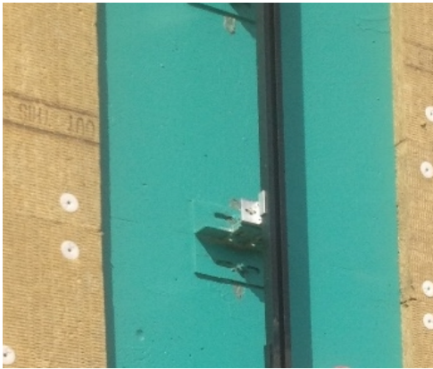
Figure 17: Example of heavy-duty engineered anchor consisting of large welded steel plates and vertical rail system.
