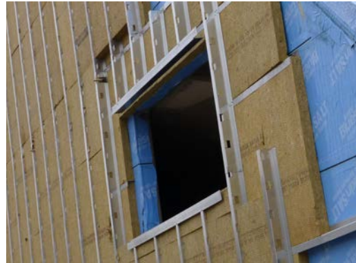
Figure 7: Crossing Z-girt cladding support system with custom punched vertical Z-girt profiles used to retain exterior insulation.
