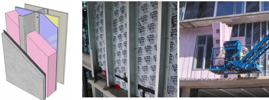
Figure 4: Vertical Z-girt over steel stud wall assembly. Girts are fastened to studs behind at every 16" o.c. resulting in significant thermal bridging through the exterior insulation.
