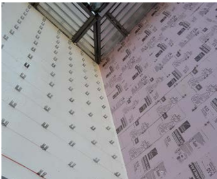
Figure 16: Examples of some different masonry ties installed through exterior insulation.
