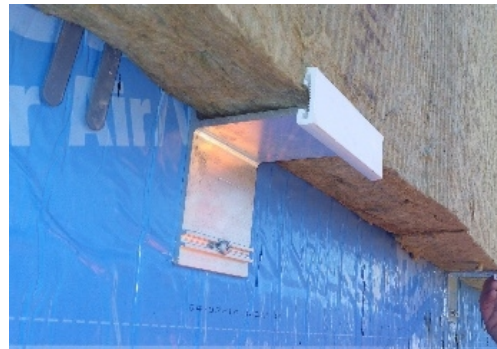
Figure 18: Examples of thermally improved discrete cladding supports for composite metal panels.
