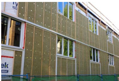
Figure 23: Example of insulation retained by mechanically attached metal impaling pins between vertical wood framing (adhesive stick-pins are not considered a long-term support strategy).
