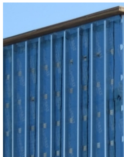
Figure 9: Intermittent galvanized steel clips with vertical girts
