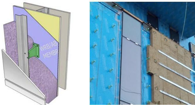
Figure 14: Fiberglass clips (spacers) attached to wall with screws, horizontal Z-girts attached to clips with screws
