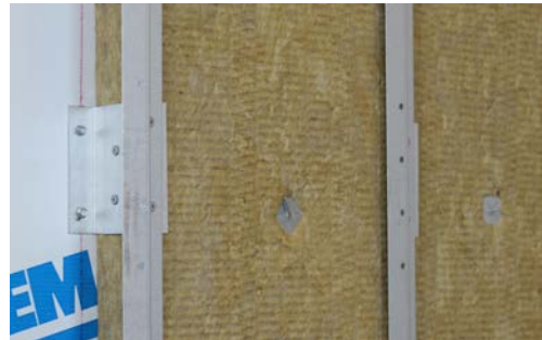
Figure 10: Generic adjustable back to back L-angle clips
