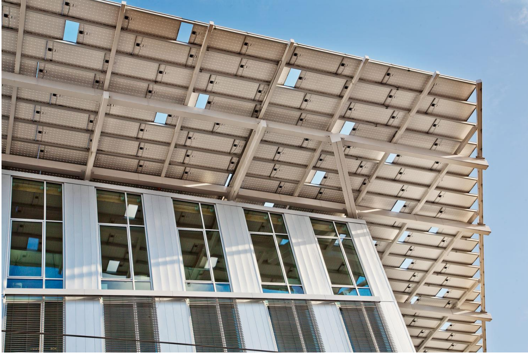
Figure 7: The Bullitt Center PV panel roof.
