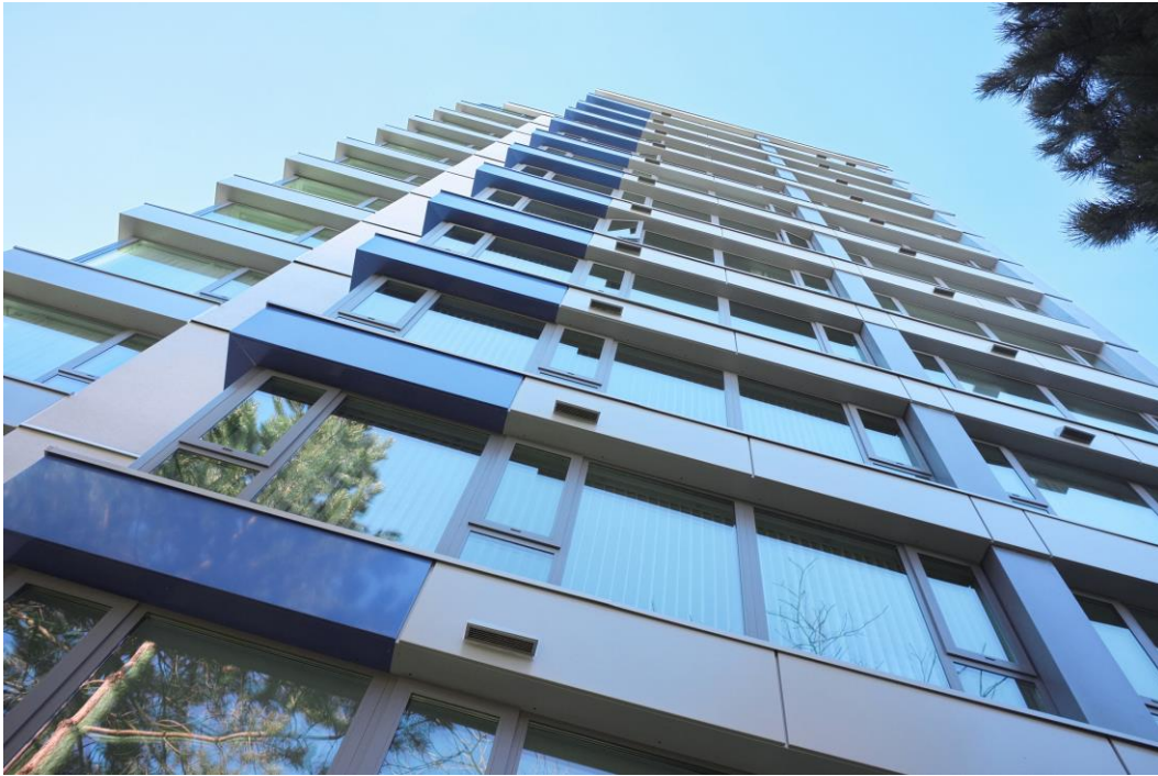
Figure 1: The Belmont Multi-unit Residential Building Retrofit in Vancouver, BC.
