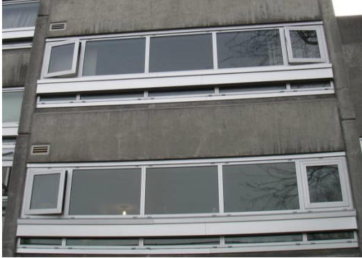
AFTER: New windows installed.
