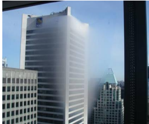
Figure 6: Volatile fogging between panes of glass occurring during periods of warm weather in direct sunlight.
