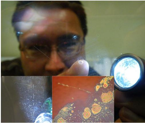
Figure 5: The author examining hazing that could not be cleaned from the glass (corrosion of silver low-e coating inside the IGU).
