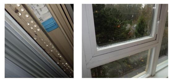
Figure 7: Condensation and mold growth on interior window surfaces
