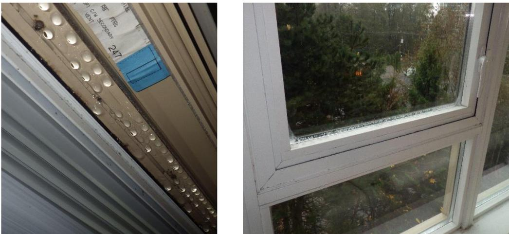
Figure 7: Condensation and mold growth on interior window surfaces
