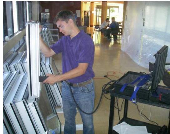
Figure 10: Testing IGU units – prior to installation
