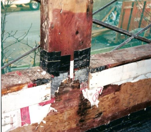
Figure 4: Membrane used at saddle detail
