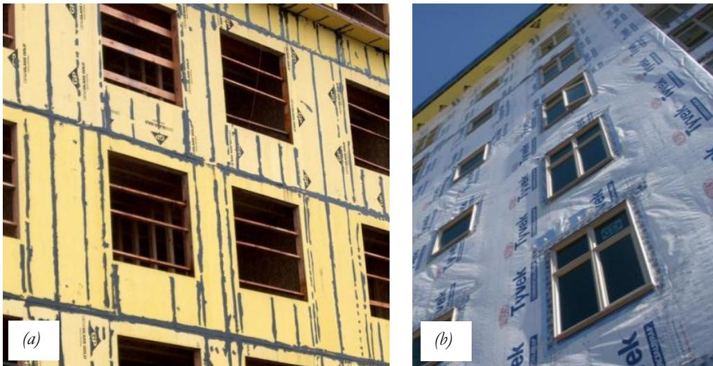
**Figure 1** (a) Sealed sheathing, prior to sheet membrane (water resistant barrier) installation. (b) Sheet-applied air barrier sealed with tape.
