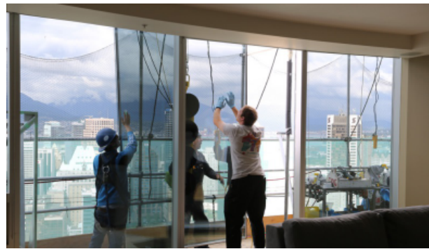
Figure 15: The IGU is positioned in the window opening.
