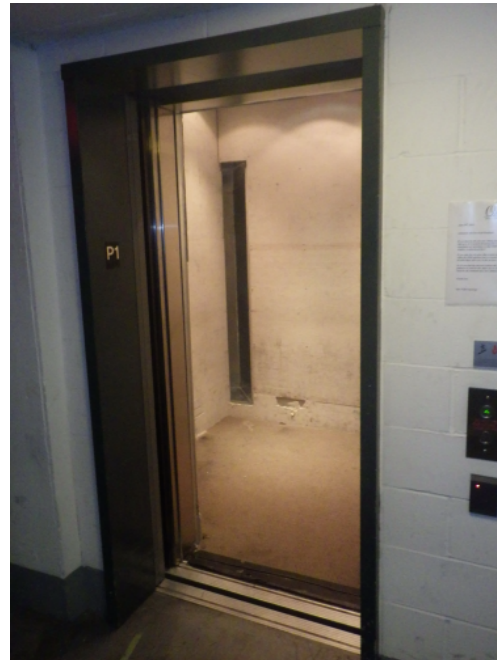
Figure 13: Completed steel notch and protection board within the elevator to protect finishes.
