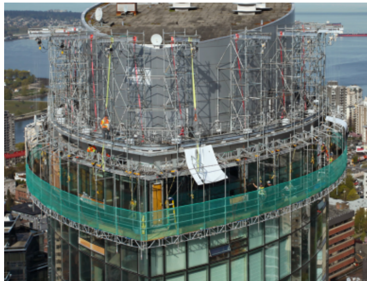
Figure 11: Installed suspended scaffolding and hoist towers
