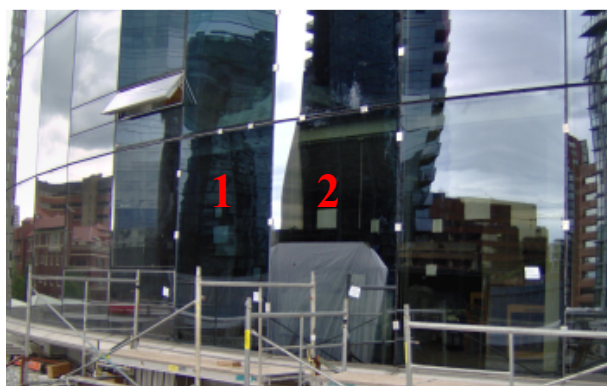
Figure 5 : Five full scale mock-ups installed at the lower hotel floors for colour comparison.
