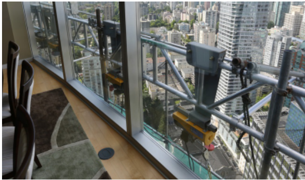
Figure 14 : IGU hoist motors mounted on the suspended scaffolding rail.
