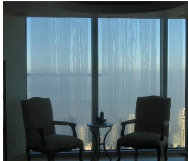
Figure 2: Fogging and corrosion of the low-e coating due to condensation within the IGU.
