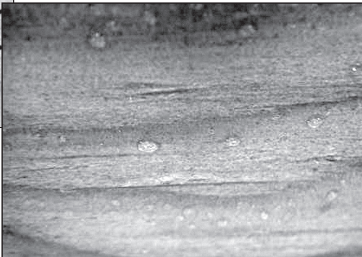
Figure 18 – Condensation on underside of plywood sheathing on the morning of January 2, 2013. Note that surface condensation at this time only occurred on certain areas of the plywood and was affected by wood grain.
