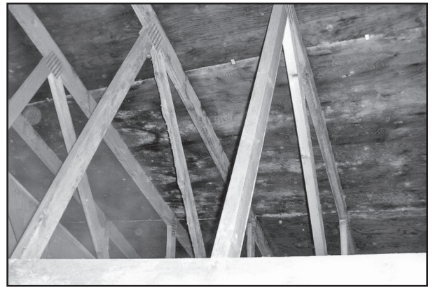
Figure 2 – A wood-frame attic with widespread stained, wet, and deteriorated sheathing from persistent indoor and exhaust duct air leakage and poor attic ventilation.
