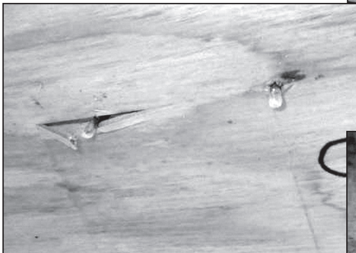
Figure 17 – Frost on nail heads of south-facing roof slope on the morning of January 2, 2013.
