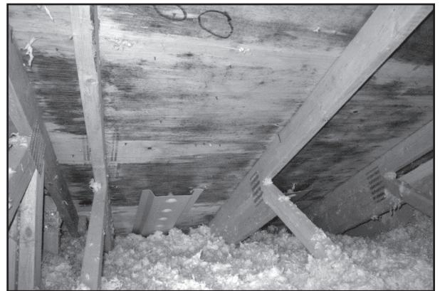
Figure 4 – Stained and damp sheathing only on the north slope of a very well-ventilated wood-frame attic not obviously linked to conventional wetting mechanisms and hypothesized to be caused by night sky condensation of outdoor ventilation air. Note that the staining is more apparent on the sapwood than the heartwood.
