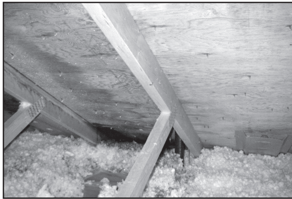
Figure 1 – Locally stained and wet sheathing and frost due to condensation of humid air leaking from a poorly sealed bathroom exhaust fan and duct.
