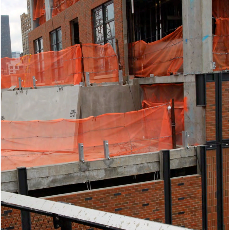
Figure 6: Identification – Veneer panels during installation.
