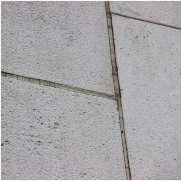
Figure 1: Identification – In a face-sealed system, there will be no visible drainage holes or tubes in the exterior sealant and no visible flashing components between panels. The sealant shown on the left is clearly failing. The photo to the right shows acceptable sealant.
