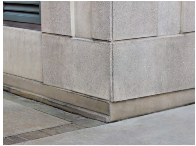
Figure 11: Chipping of panel edges. Physical impact can lead to damage to panel edges, especially at corners (as pictured on left), and where the concrete has been formed into a sharp edge for aesthetic or functional reasons. Careful patching and cleaning, as shown in the photo on the right, can fix such damage.
