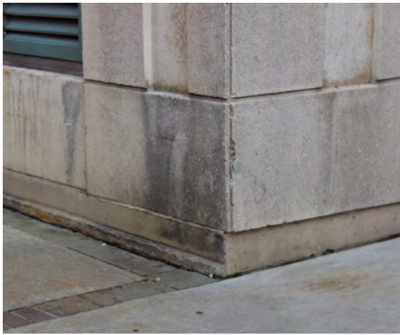
Figure 11: Chipping of panel edges. Physical impact can lead to damage to panel edges, especially at corners (as pictured on left), and where the concrete has been formed into a sharp edge for aesthetic or functional reasons. Careful patching and cleaning, as shown in the photo on the right, can fix such damage.
