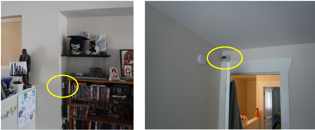
Figure 2.4 Temperature, relative humidity, and CO2 sensors installed in Unit 5
