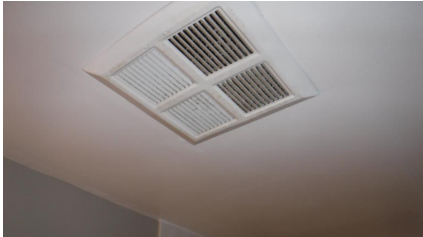
Figure 1.9: Bathroom exhaust fan unit. Air from the interior space can enter the exhaust duct due to the combination of wind, stack effect, and mechanical pressures, where it can then cool and condense.
