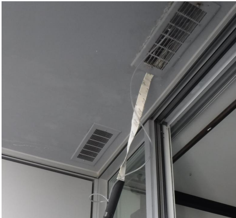
Figure A.11: Photo of the sensor installation at Site C. Dryer exhaust vents under the exposed concrete balcony of the unit above.
