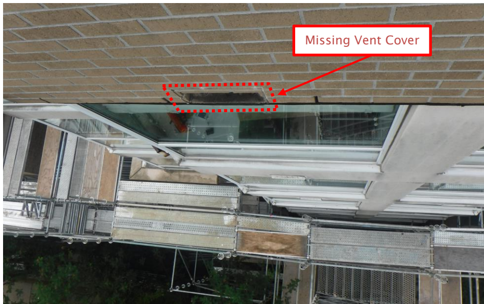
Figure 1.10: Photograph taken of a wall from above showing an exhaust vent opening. Note the vent cover has been removed and the duct is therefore exposed to rainwater.
