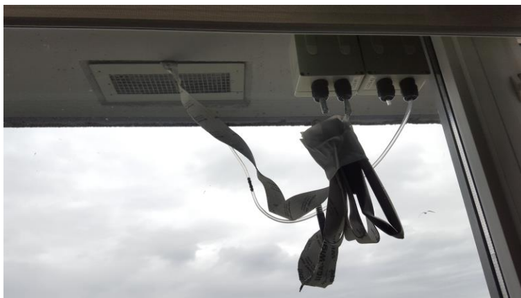
Figure A.2: Photo of the sensor installation at Site A. Dryer exhaust vents under a soffit.
