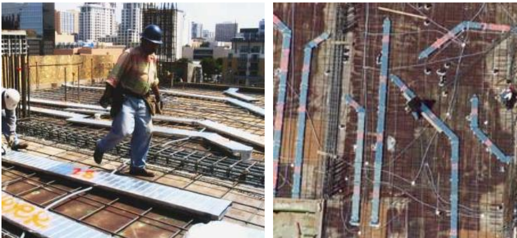
Figure 1.1 Installation of in-slab ducts.
