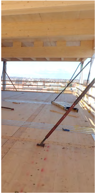
Figure 14 Splice joint and drag strut connections visible at CLT panel interfaces.
