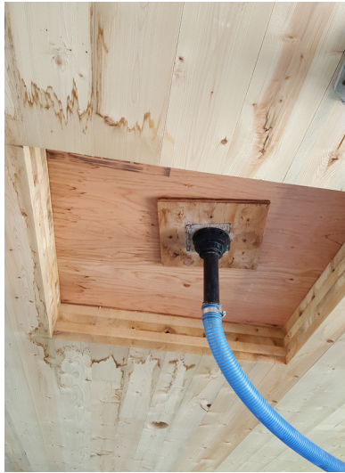
Figure 22 A temporary drain connection at a mass timber roof panel.
