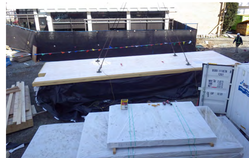
Figure 13 A CLT floor panel with a factory-installed membrane is being hoisted into place at a project site.
