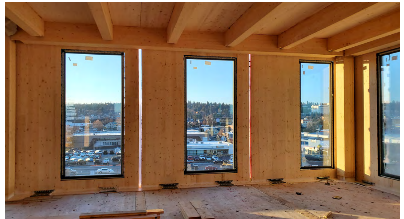
Figure 21 CLT wall panels with factory-installed air barrier and WRB membrane and window rough opening membranes prior to on-site installation of windows and panel joints.
