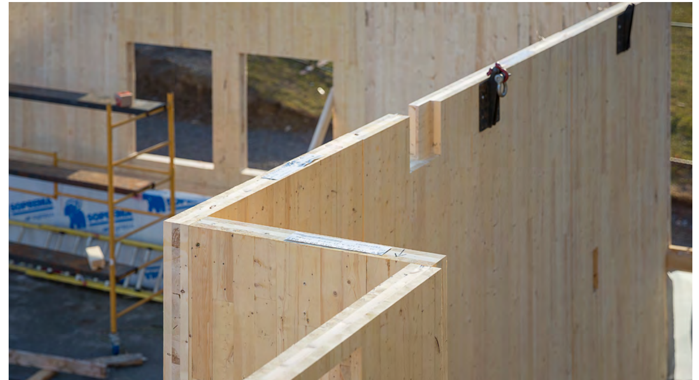
Figure 20 CLT wall panels with exposed penetrations and rough openings prior to on-site application of a WRB membrane.
