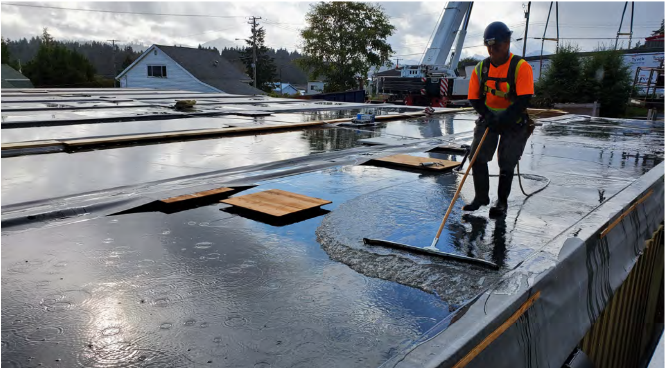
Figure 23 A worker removes standing water from a wood-framed roof assembly using a squeegee.
