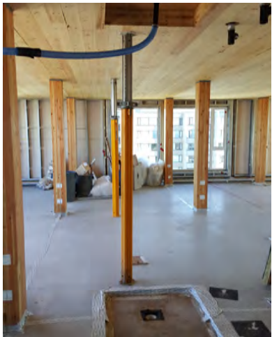
Figure 7 Mass timber floor assembly with cementitious topping.
