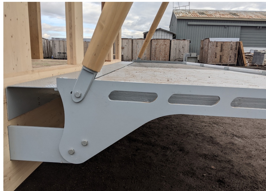
Figure 23 A custom steel connection provides intermittent attachment of the balcony element to the wall, reducing thermal bridging across the exterior wall insulation (not shown) at the interface.
