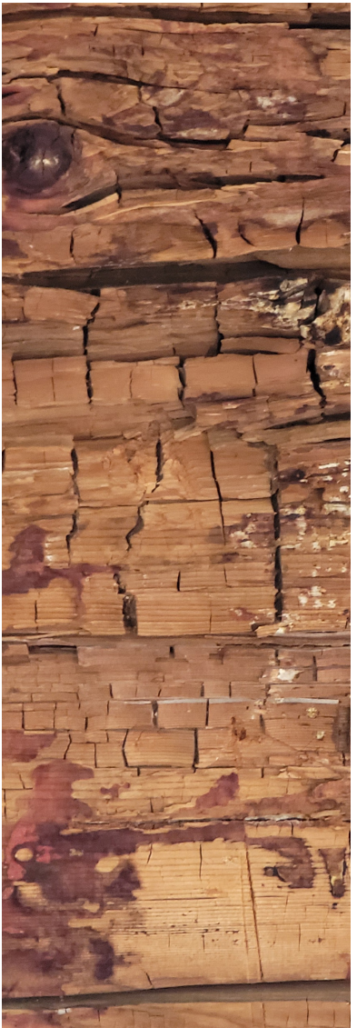
Figure 3 Decomposition of a CLT floor panel caused by an impermeable membrane trapping moisture in the wood and preventing drying.
