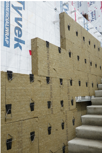
Figure 10 In-progress installation of exterior mineral wool insulation.
