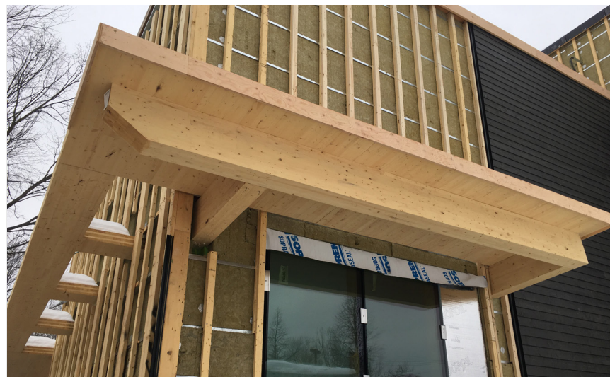
Figure 31 Vertical strapping installed over exterior insulation to create a drainage cavity in the rainscreen wall assembly.
