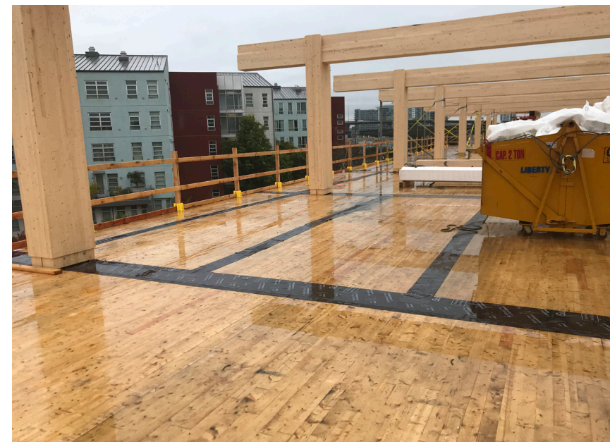
Figure 5 CLT floor assembly exposed to moisture during construction.
