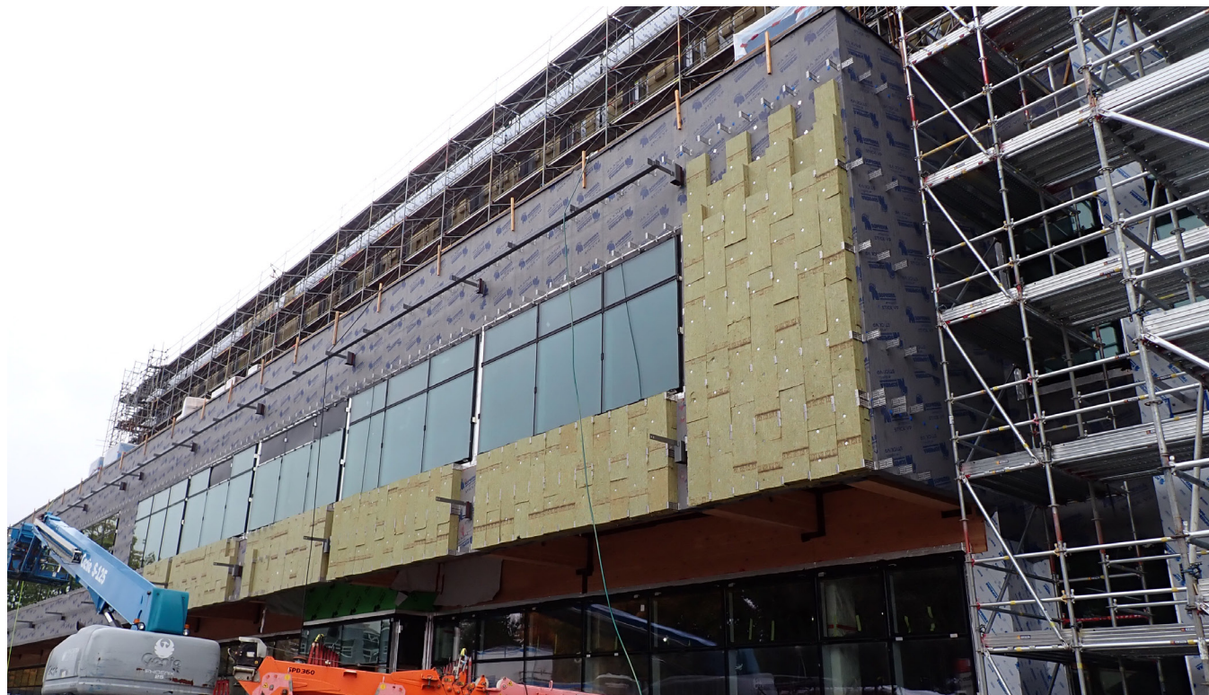
Figure 13 A clip and rail cladding attachment system and mineral wool insulation make up the thermal control layer of the mass timber wall assembly on this building.
