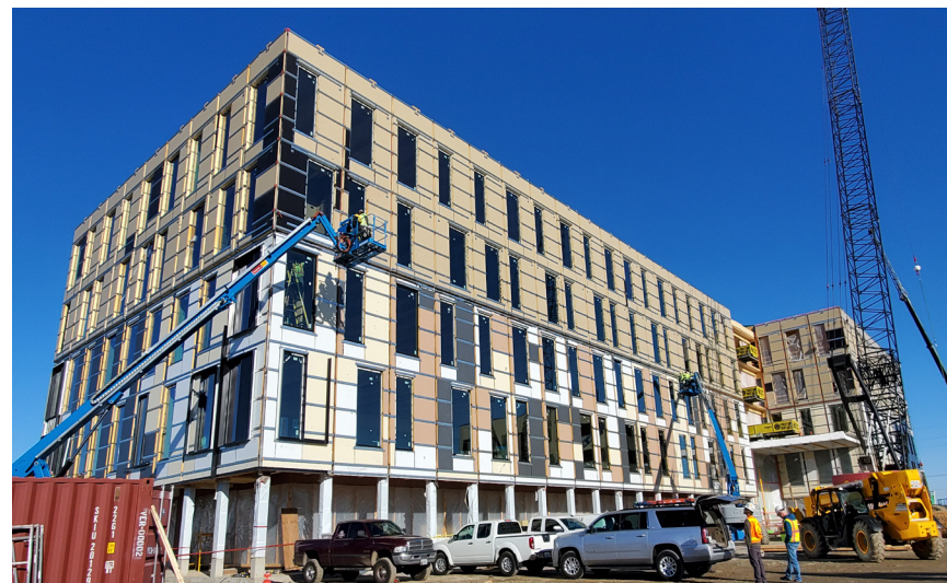
Figure 33 Rigid insulation located exterior of the mass timber walls.
