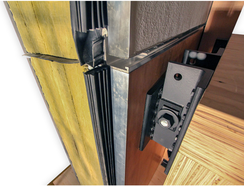
Figure 22 A horizontal stack joint concept at a panel-to-panel connection shown on a super-insulated wall assembly mock-up.
