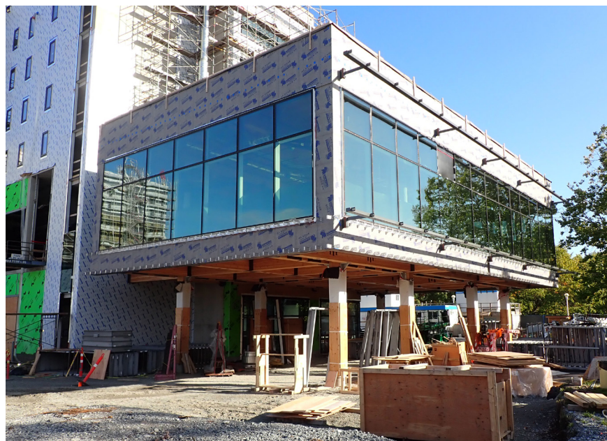
Figure 7 A fully adhered air barrier and WRB membrane over a mass timber wall substrate.
