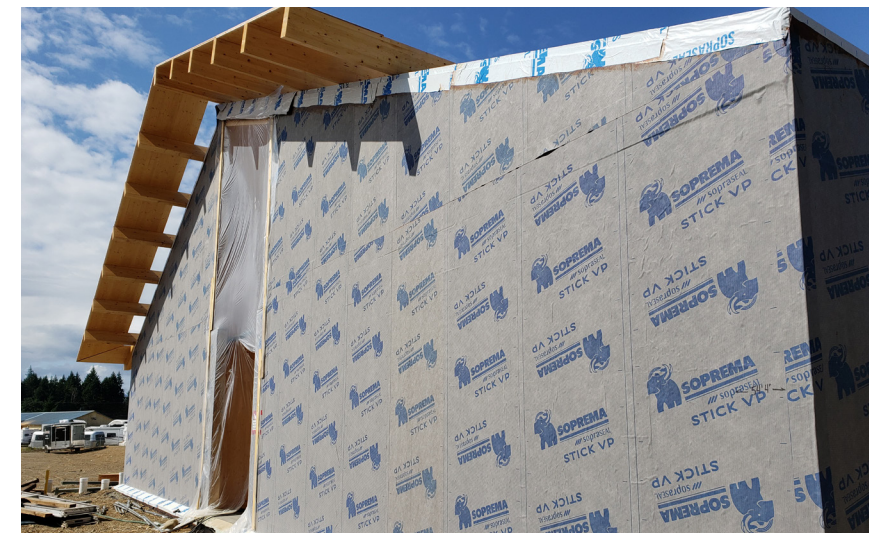
Figure 32 In-progress installation of a self-adhered vapor-permeable air and WRB wall membrane. The wall membrane is continuous with the air barrier membrane at the roof.
