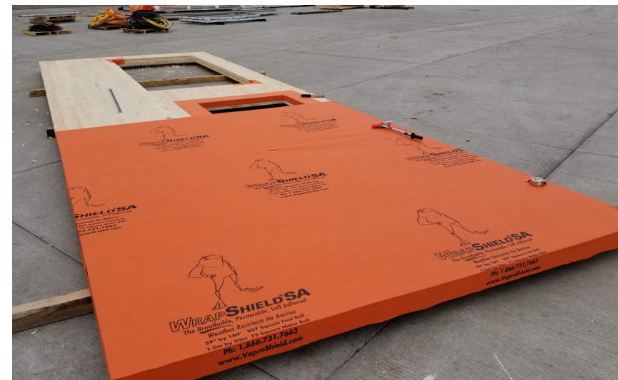
Figure 34 Vapor-permeable self-adhered air barrier and WRB membrane installed on a mass timber prefabricated panel while at the factory.
