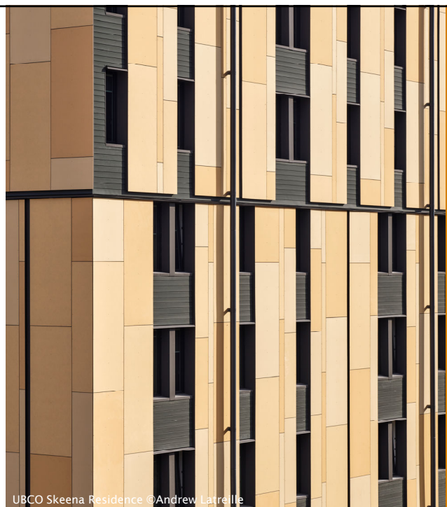
UBCO Skeena Residence ©Andrew Latrelle
