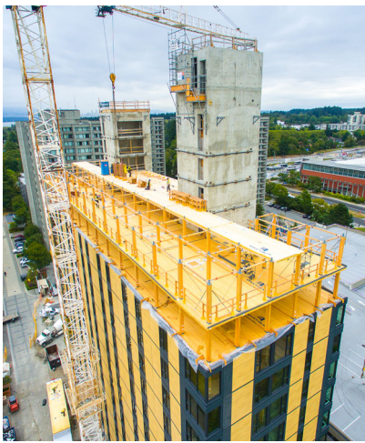
Brock Commons by Acton Ostry Architects ©Naturally Wood
