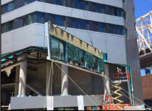
Prefabricated metal wall panel installation
