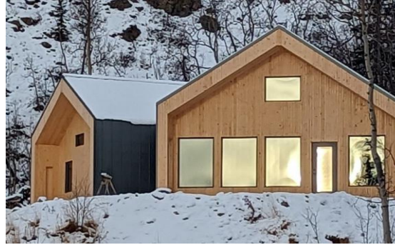
Figure 11: The triple-glazed, double low-e coated windows installed in the case study building. The south elevation has SHGC 0.48 windows to maximize the solar heat gain, while other elevations have SHGC 0.28 windows.
