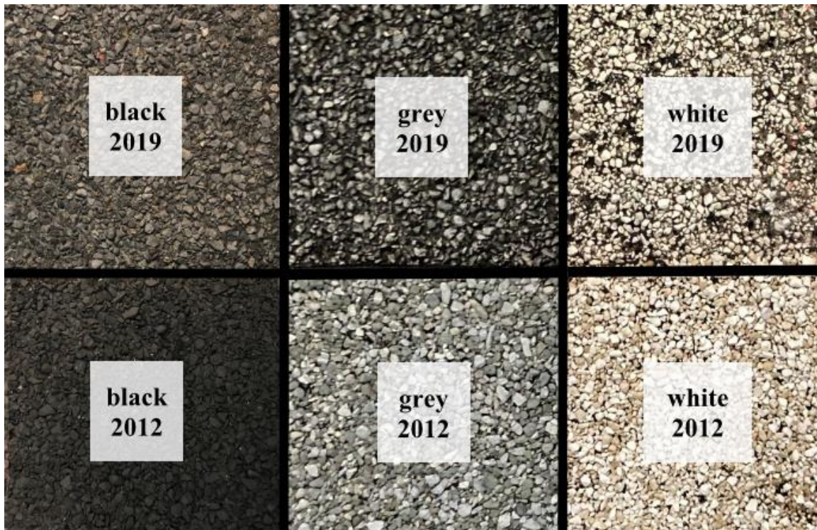
Figure 7 - Roof membrane samples comparing original 2012 vs. aged 2019 for black, grey and white membrane color.
