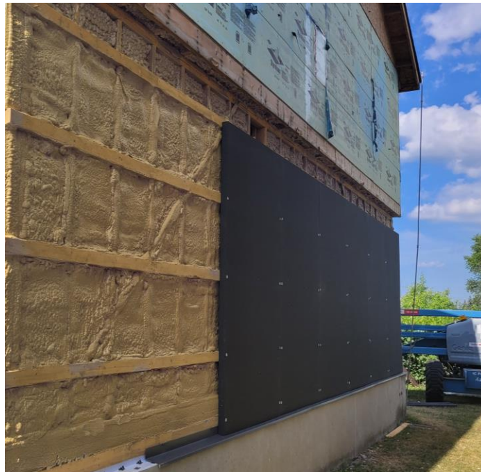
Figure 3: BASF first-floor insulation in progress (second floor is original).
