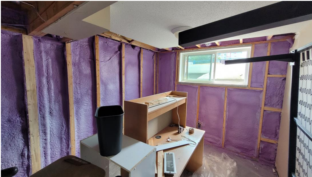
Figure 8: Spray foam installed against the interior of the foundation wall.
