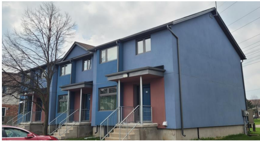
Figure 4: Dryvit wall system with finished EIFS deep energy retrofit enclosure.
