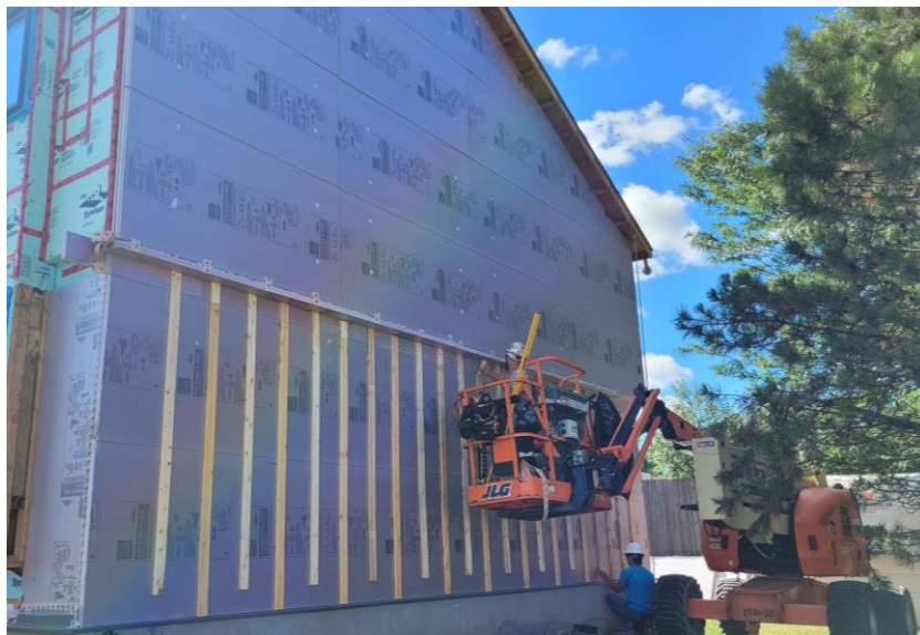
Figure 5: Owens Corning exterior insulation being installed with strapping.
