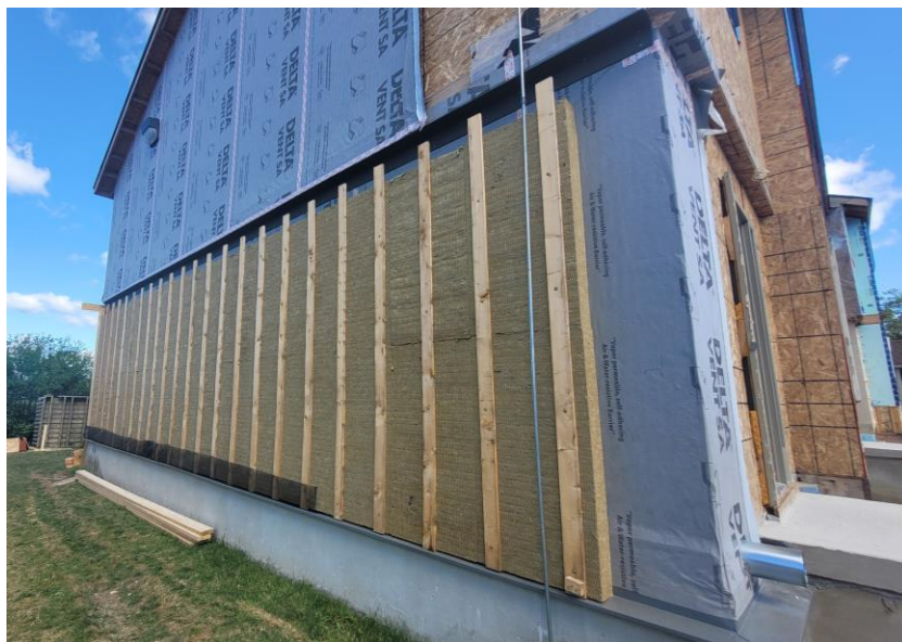
Figure 7: ROCKWOOL deep energy retrofit wall assembly.
