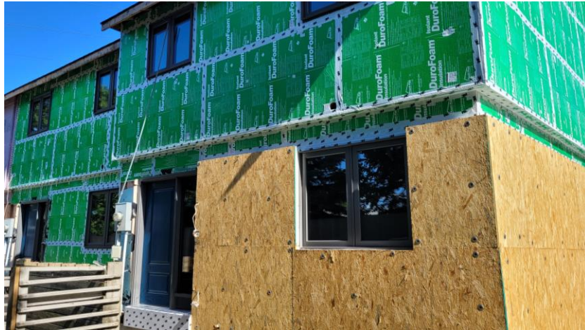
Figure 6: Plastifab Insulspan deep energy retrofit wall assembly during installation.
